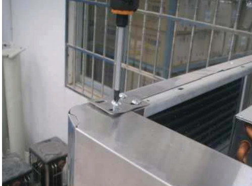
A. Disassemble the top grille fixture as below.
