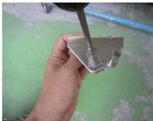
C-2. Disassemble bottom hinge (left).
