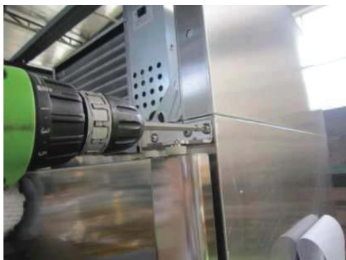
A. Unscrew screws located on top hinge (right).
